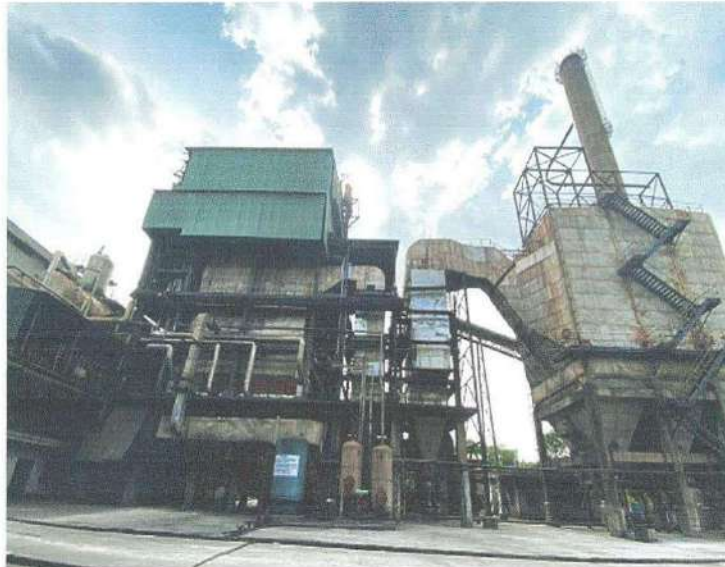
Bag filters Attached with Chimney – Ferro Alloy Plant
