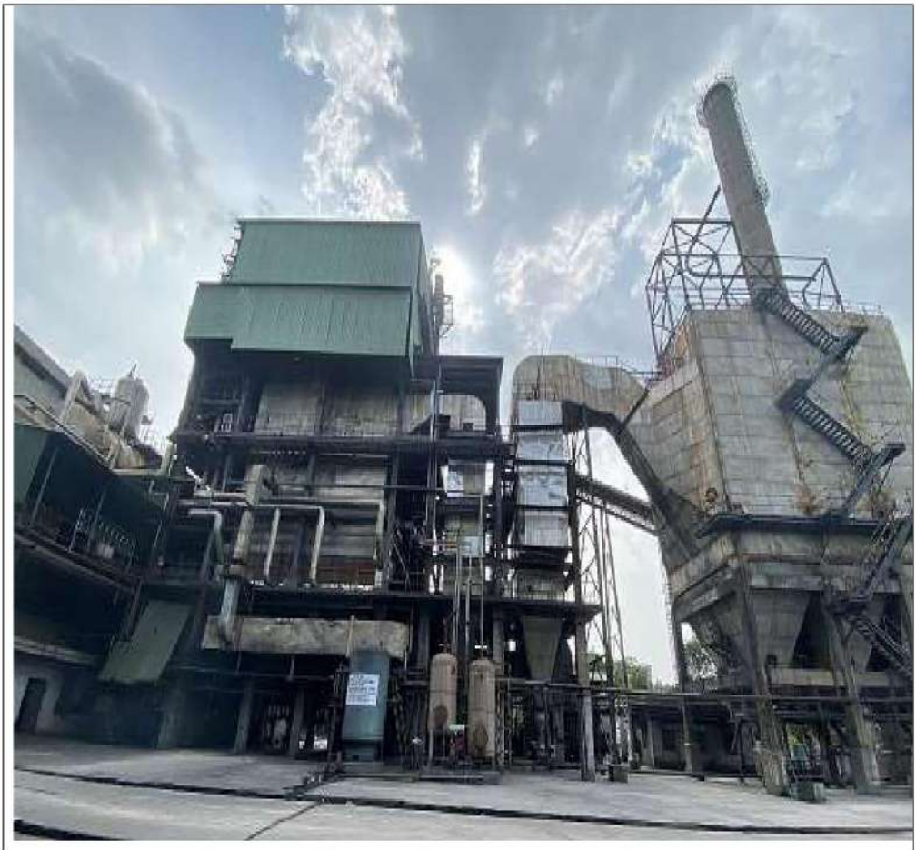
Bag filters Attached with Chimney – Ferro Alloy Plant
