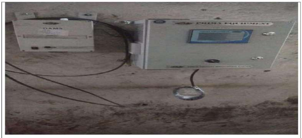
Online Gas Analyzer for continuous emission monitoring at Chimney – Power Plant
