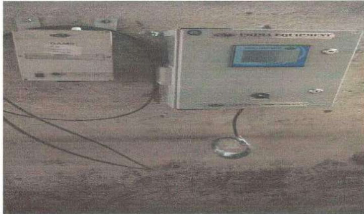
Online Gas Analyzer for continuous emission monitoring at Chimney – Power Plant
