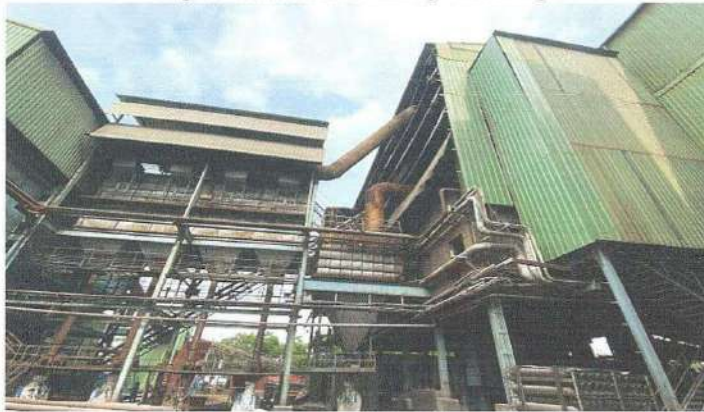
Bag filters Attached with Chimney – Ferro Alloy Plant
