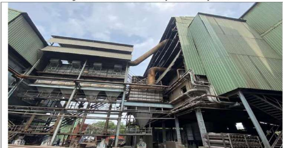
Bag filters Attached with Chimney – Ferro Alloy Plant
